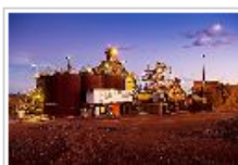
The Gullewa gold project
